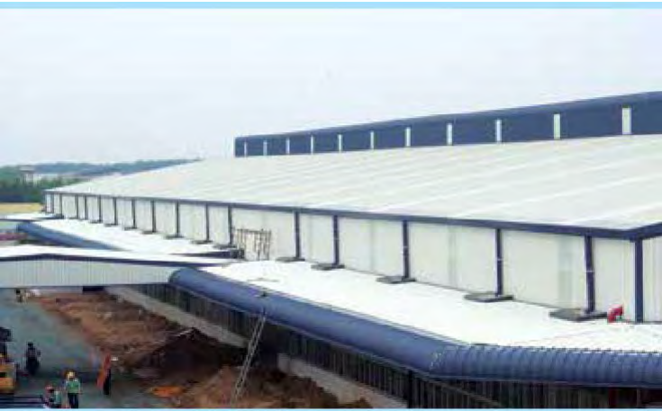
Beesco Vina Binh Phuoc - Water Distribution Tray
