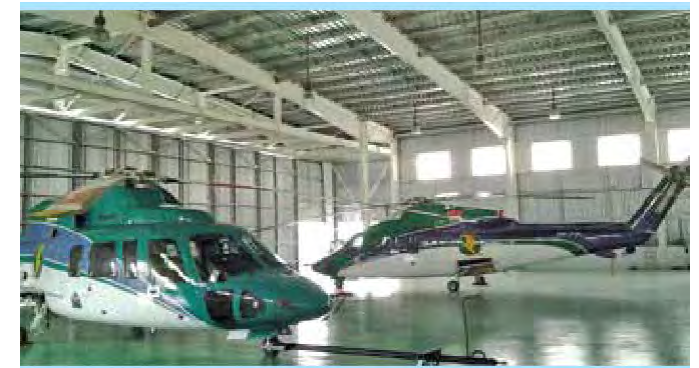
Helicopter Hangar (Myanmar)
