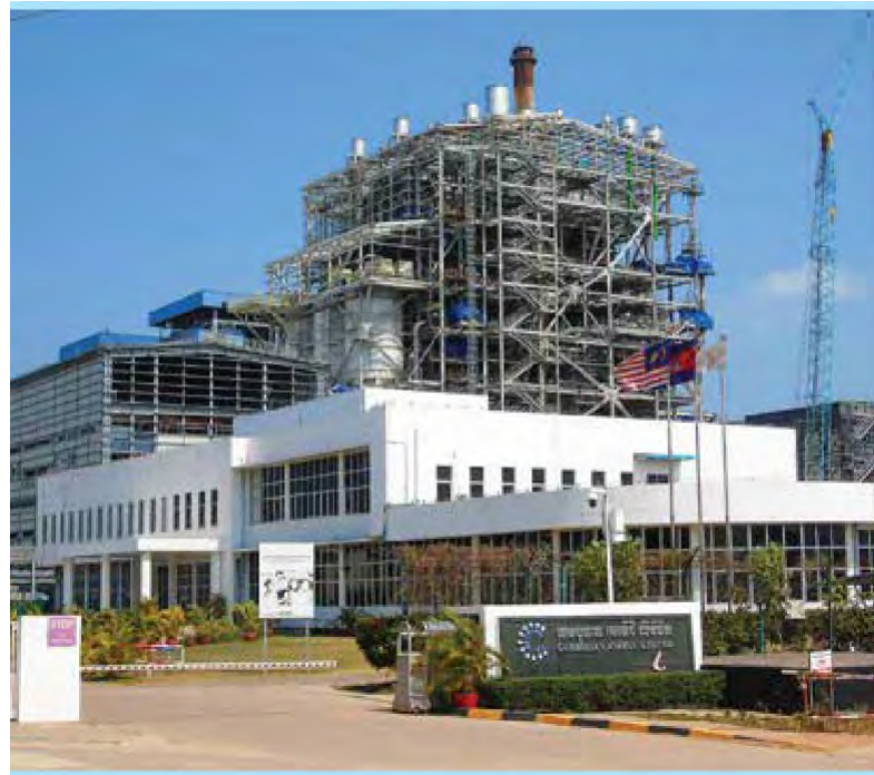
Narawat Power Plant (Cambodia)
