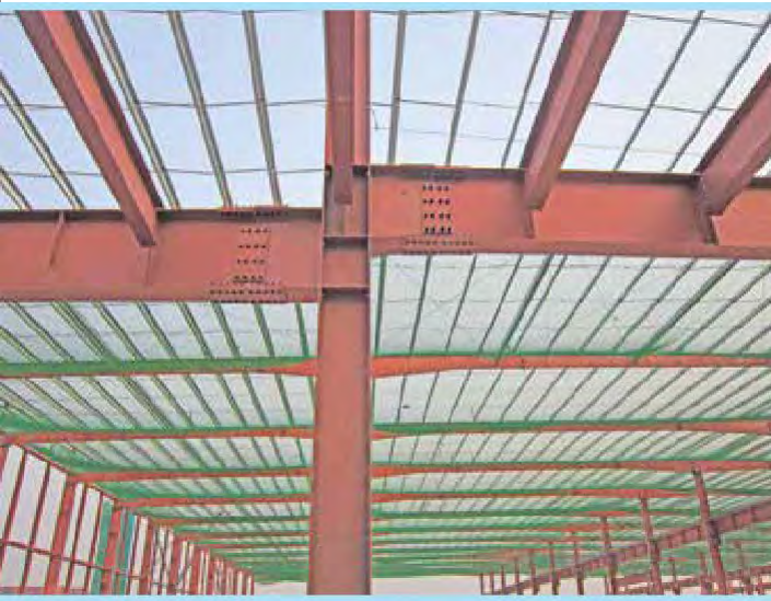
LG Electronics Haiphong Factory (GS - Serve One) - 1,620 MT
