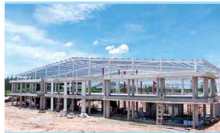
Ticon Logistic Warehouse (Thailand)
