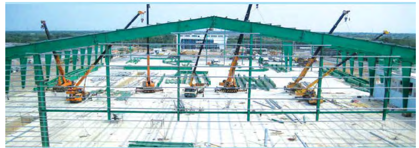
90M Clear Span for California Waste Solution (USA) ---1,320 MT
