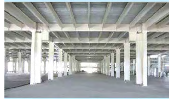
Mezz: Column, Beam, Joist, Deck
