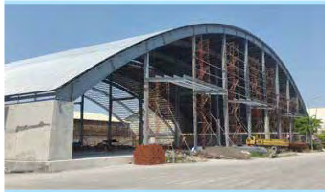
NPK Warehouse, Wilmar Project (Indonesia)
