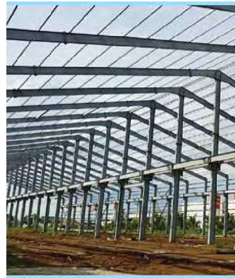
SJC Concrete Warehouse (Thailand)
