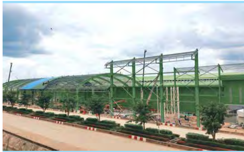
FCB Warehouse Phase 2 (Thailand)
