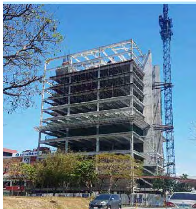
14-floor Workspace Building (Philippines)
