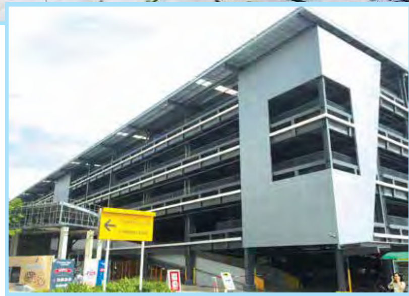
Four - Floor Parking of Aeon Mall PhnomPenh, Cambodia
