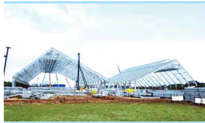
Flat Storage, Krakatau Bandar Samudera, Cilego (Indonesia)
