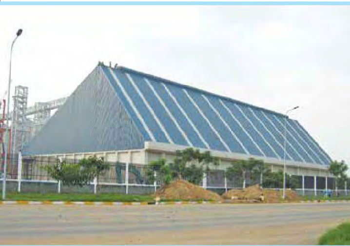
102% Roof Slope, SoyBean Meal Factory (Baria Serece)
