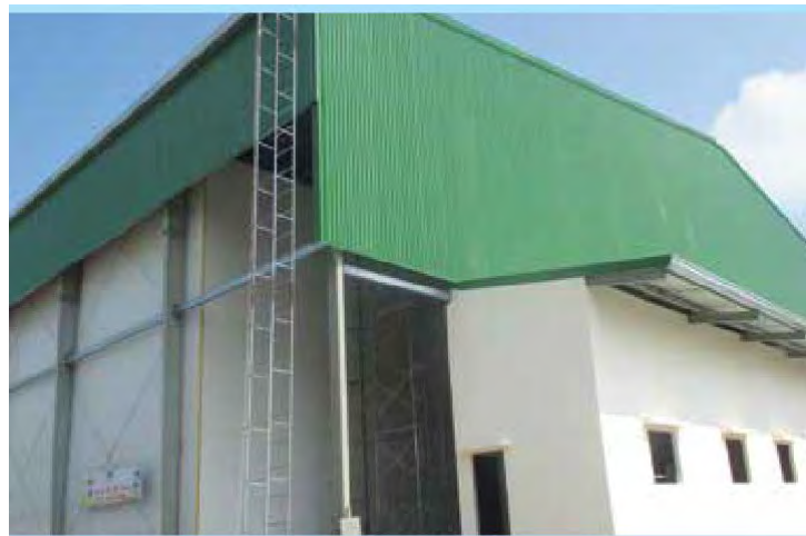
Truong Giang Fishery Cold Storage (Panels Inside Columns - GMP License)
