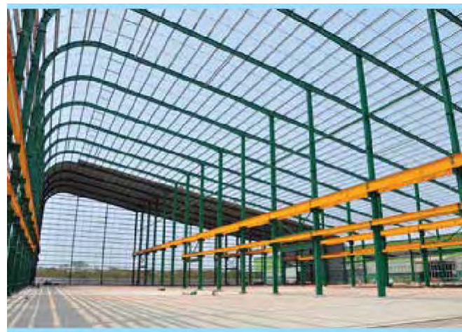
Permsin Steel Factory (Thailand)
