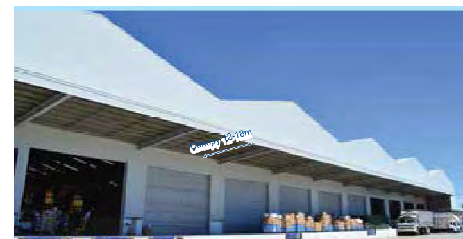
BonPack Warehouse (Philippines) (Loading bay with huge wide canopy of 12-18m)
