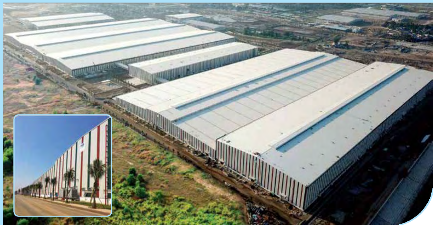
VinFast Automobile Manufacturing Complex (Haiphong - Vietnam) - 14,000 MT
