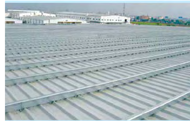
Composite Roof with Sub Purlin
