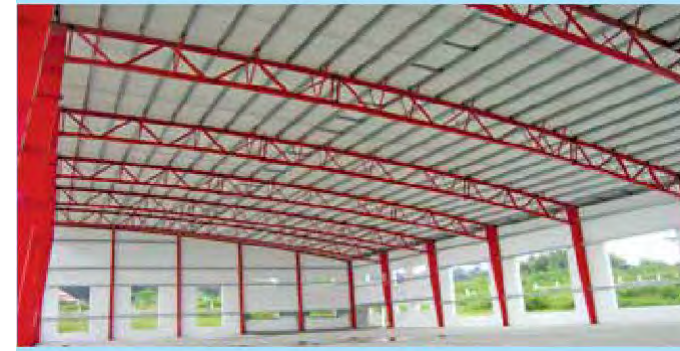
Jade Land Warehouse (Myanmar)
