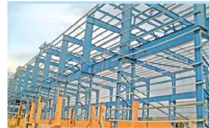
Steel Pipe Factory (Nippon Steel - Japan)
