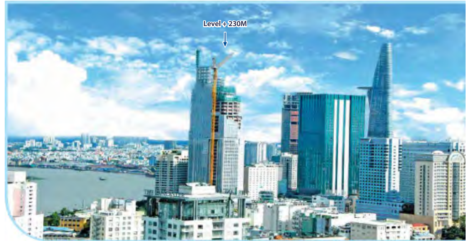
230m High, Top Roof Steel Structure for Vietcombank Tower
