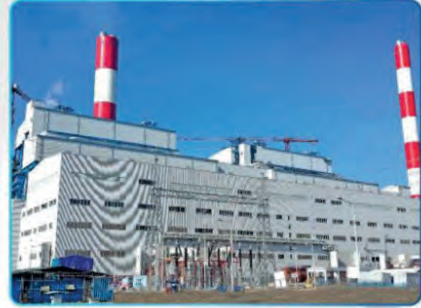
Siding Works Project of Mong Duong II Power Plant (Doosan) - 50,000m 2
