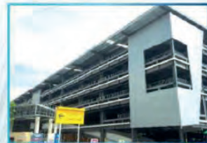
Four - Floor Parking of Aeon Mall Phnom Penh, Cambodia
